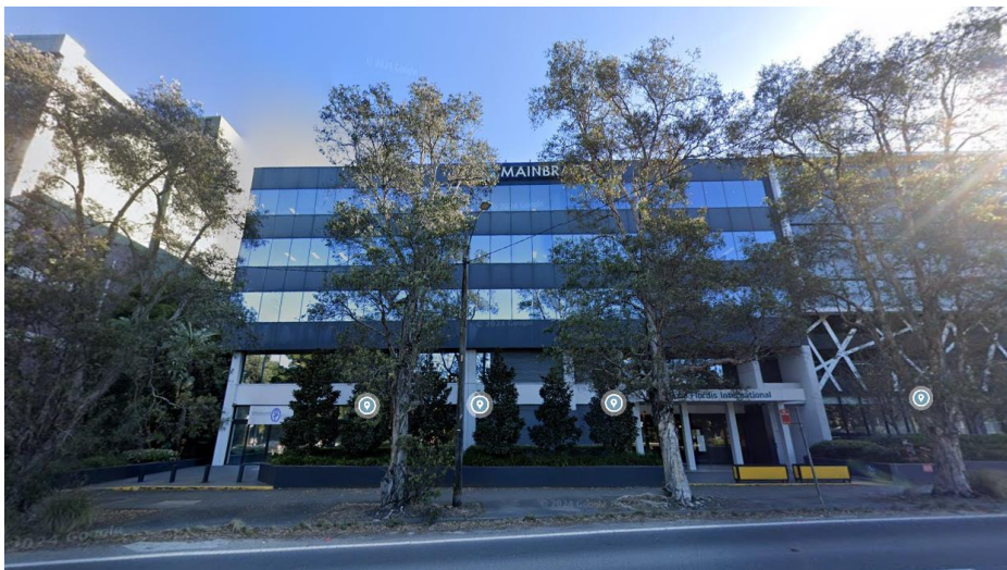
Photograph #1: Shows 170 Pacific Highway, Greenwich (Photo courtesy of Google Street View)
